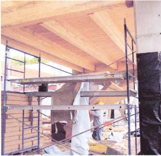
ROOF DECK GOING UP
