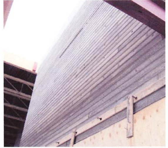
THE WESTLAND-BUILT CONCRETE FEATURE WALL
